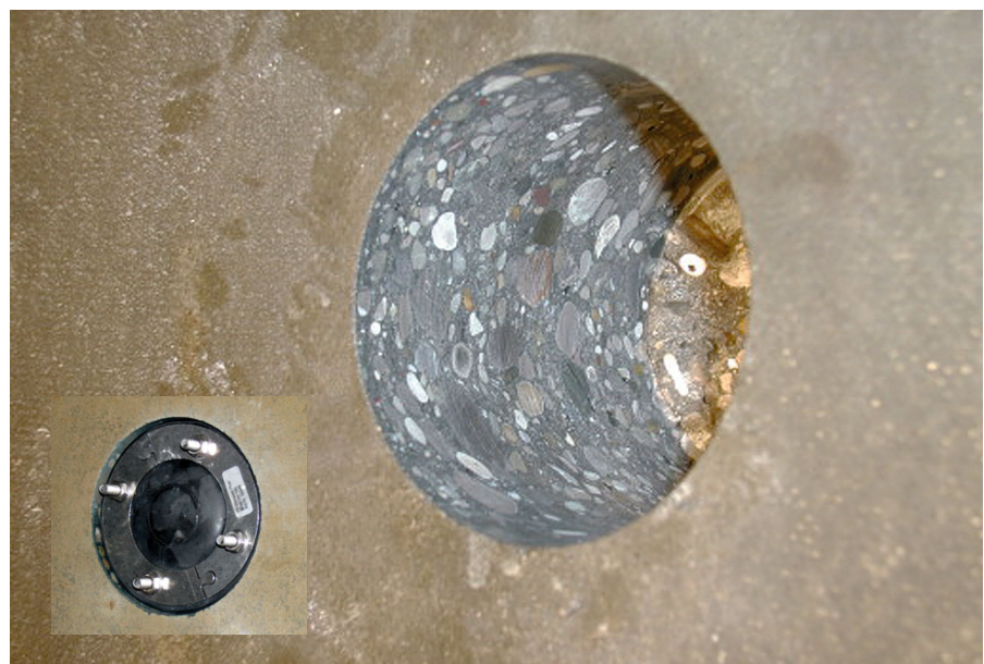
Figure 5: Borehole open and borehole sealed (blind seal used)
