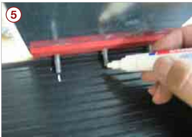
5 Position the expansion joint connector on the expansion joint waterbar and mark the required drill hole positions.
