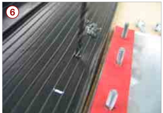
6 Drill the required holes into the expansion joint waterbar using a drill with a DN 6 mm bit.
