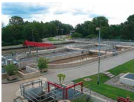
Picture 1: Reinforced concrete structures at wastewater treatment plant Bonn-Beuel exposed to high chemical and/or physical attack.
