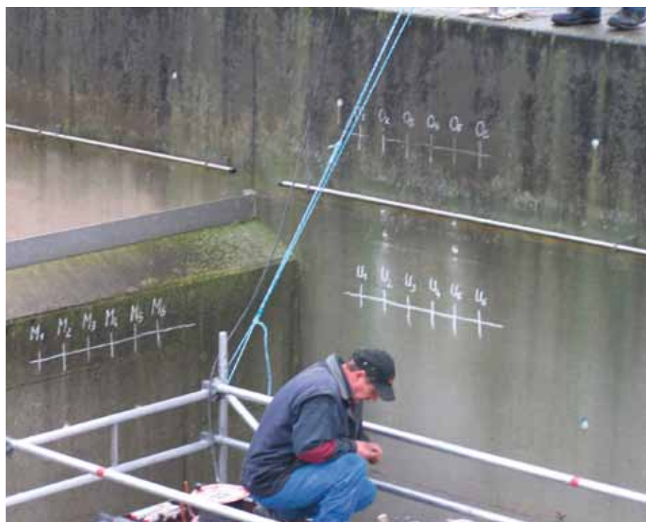
Picture 2: Offenburg-Griesheim: Core extraction locations at external wall and spillway wall
