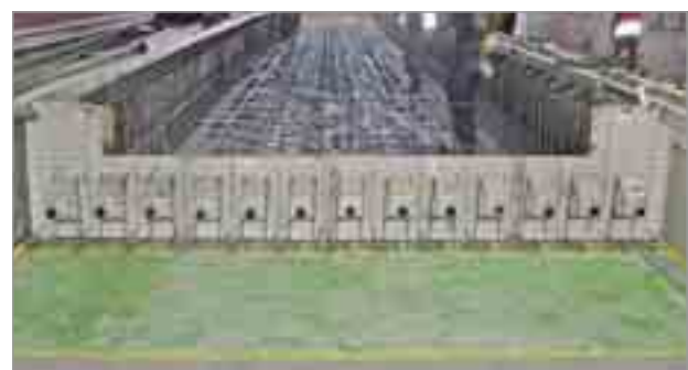
Complete formwork element combining Egcodorn and Stremaform® pre-installed and delivered onto site for expansion joint construction
