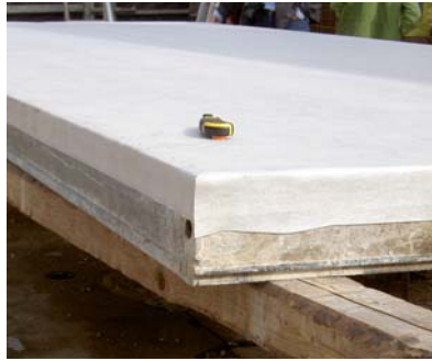
Zemdrain® MD self-adhesive fixed to the formwork
