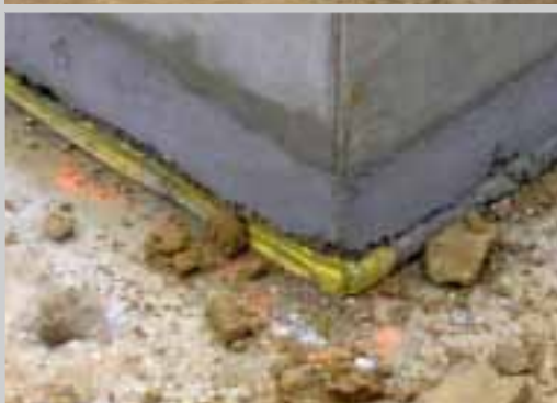
Void former (yellow) under pile head beam
