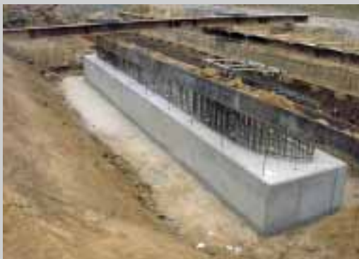
Pile head beam for central column
