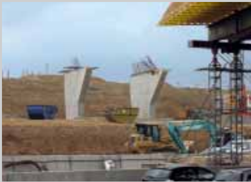
Bridge piles on a highway flyover
