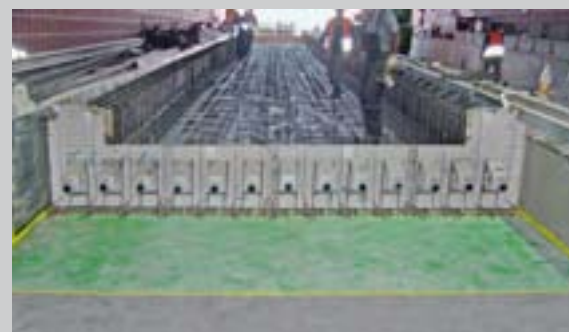
Complete formwork element combining Egcdorn and Stremaform pre-installed and delivered onto site for expansion joint construction
